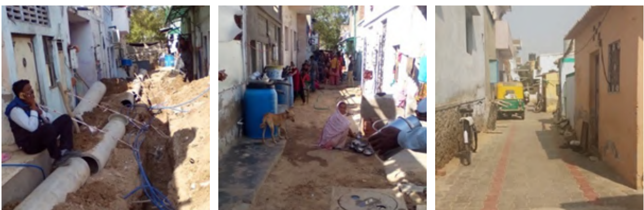
Figure 24: Stages of infrastructure construction in a street of a Parivartan settlement
